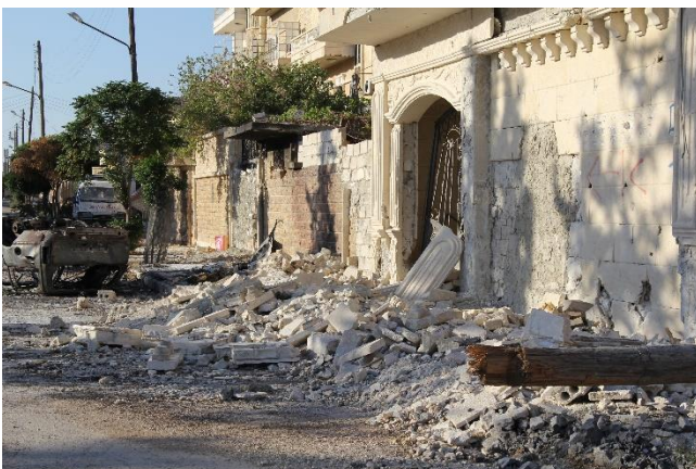
A destroyed health facility in Aleppo, Syria. Photo by Syrian American Medical Society.
