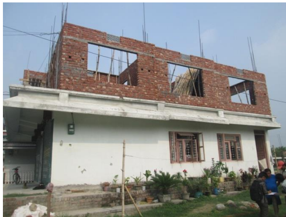
Photo: Storey being added to the existing infrastructure
