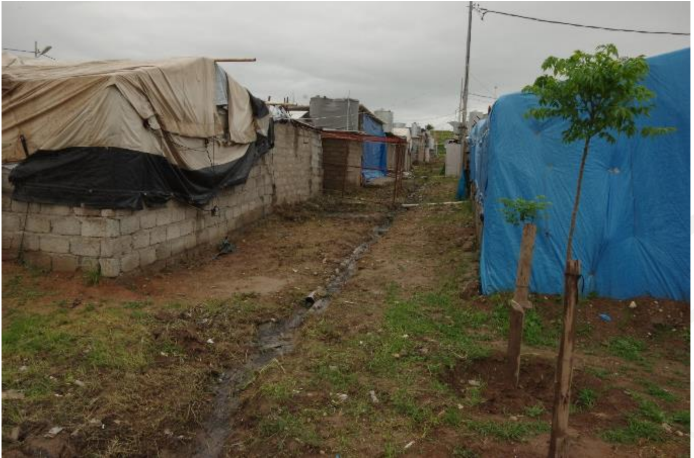
Photograph 4: greywater / wastewater surface drain from between houses in Domiz I
