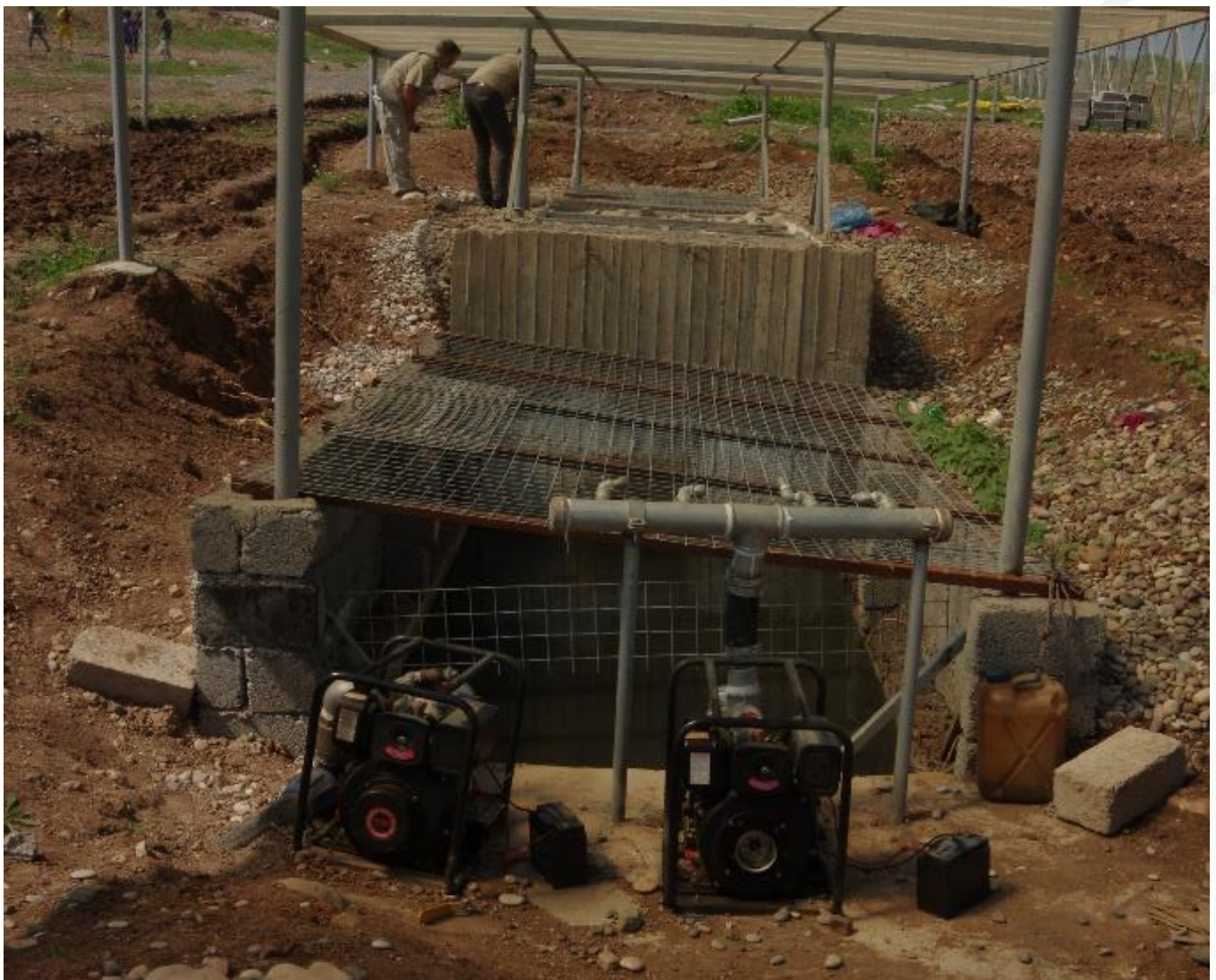
Photograph 7: the recently installed greywater treatment system in Darashakran, which uses aggregate filtration
