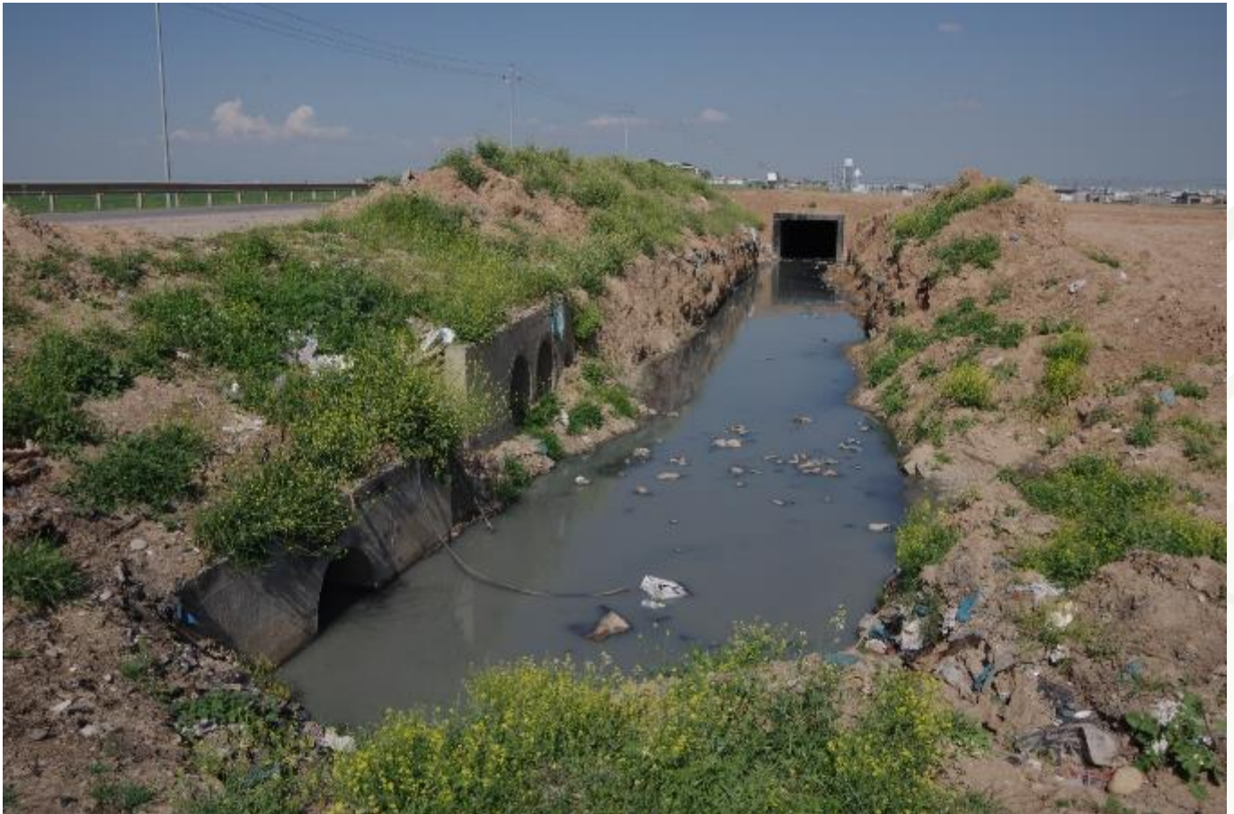
Photograph 9: the end of the extended culvert exiting Qushtapa camp (visible in the background)
