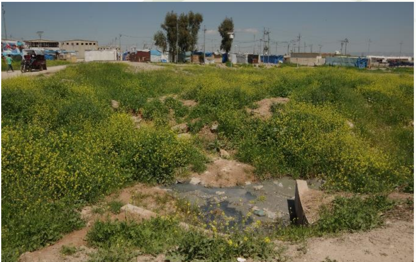
Photograph 8: the outflow of one main drainage channel at Baharka IDP camp
