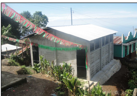
Figure 7 Constructed community hall and shelter
