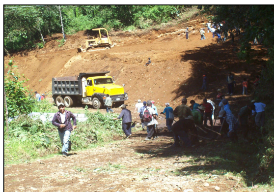
Figure 6 Access road improvement
