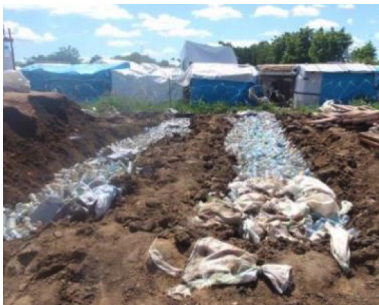
Figure 10. Shallow latrines blocked with plastic bottles. (Source: Victoria Hammond)
